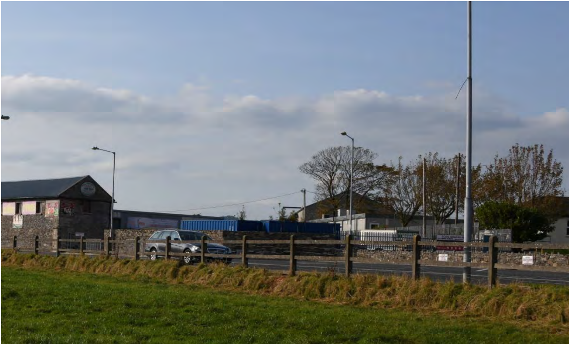
Plate 1. Road to the north of the site.
