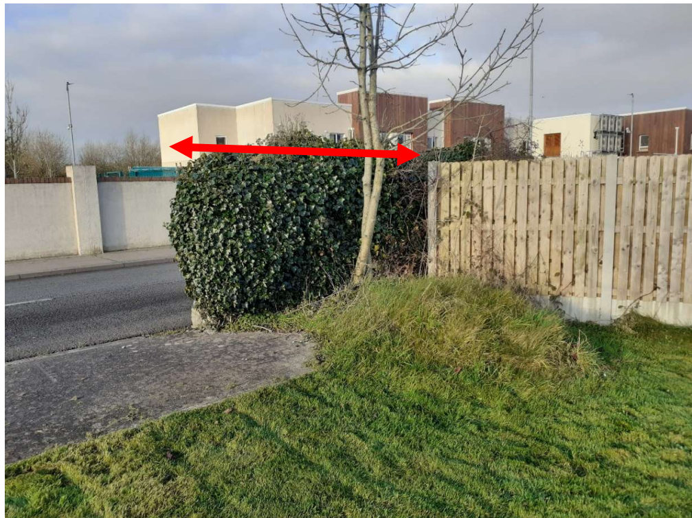
Photograph 5.3 Section of Wall, Young Ash Tree and Ivy Cover Contributing to the Sight Line Issue on Duckspool Road
