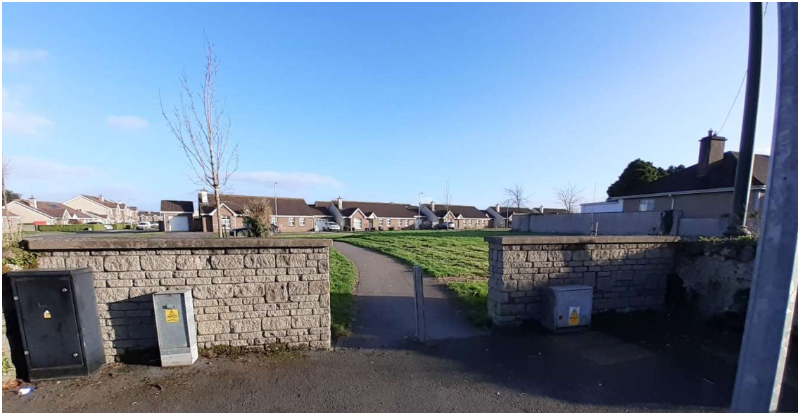
4.2 Existing N25 Entrance to Tournore Park
