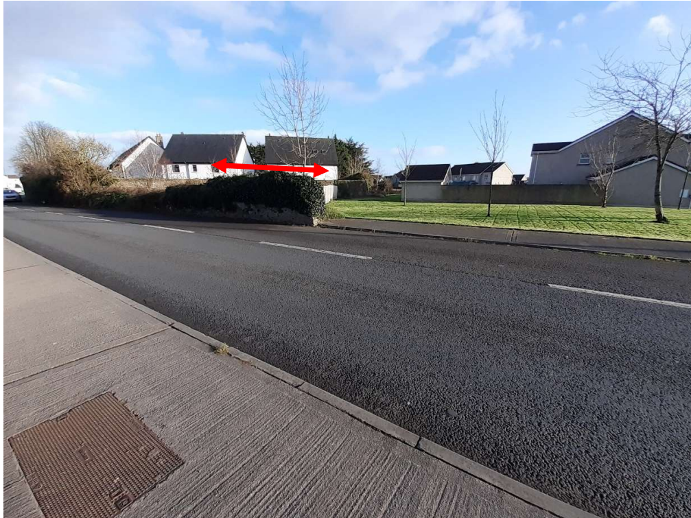
Photograph 5.2 Sight Line Issue (due to bend on Duckspool Road) for Cars Approaching the Proposed Pedestrian Crossing
