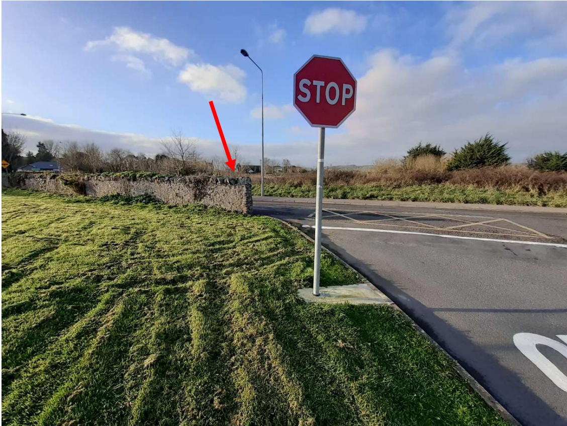
Photograph 5.4 Difficult Left Turn onto Duckspool Road Caused by Existing Stone Wall
