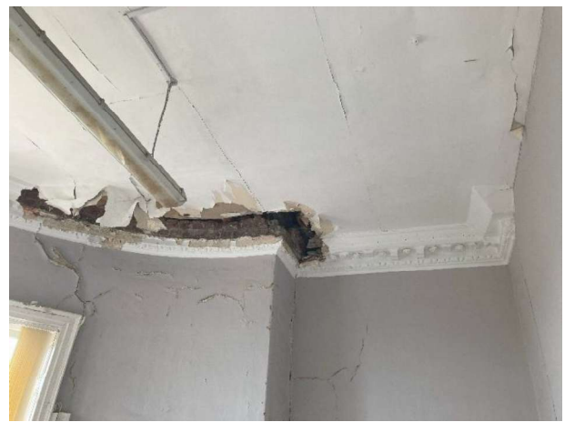
Left of chimneybreast corner detail.
