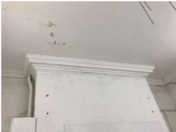
Chimney breast cornice.
