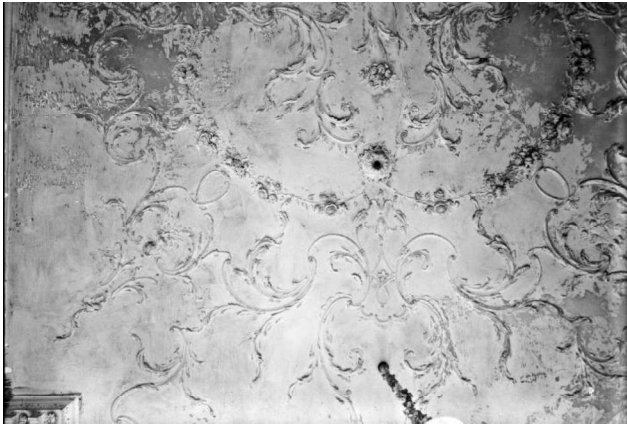
Original rococo ceiling detail.
