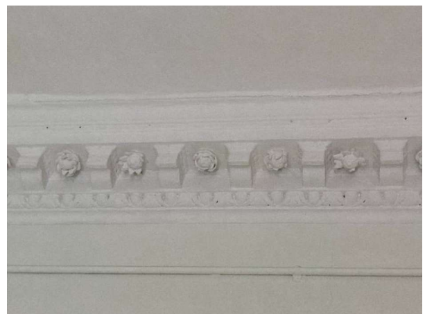
Surviving cornice detail.
