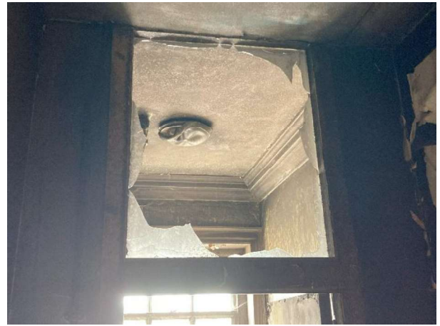
Cornice running through from 2.01-2.02.
