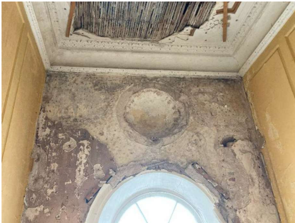
Arched window & filled niches.
