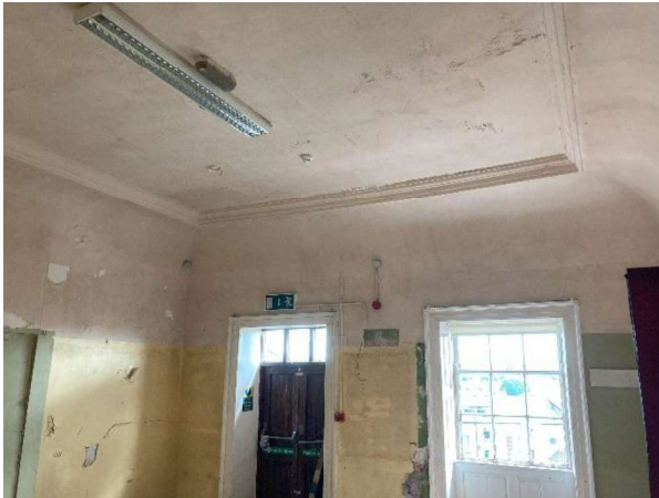
Coved detail similar to Room 2.06 but with extra run mould detail around the compartment.
