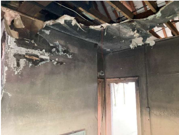
Looking east into 2.08.
