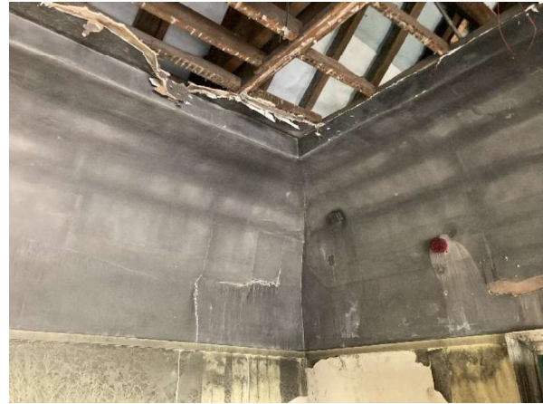
Coved detail, possible modern replacement.
