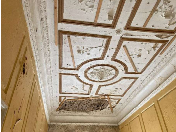
Overall view of ceiling.
