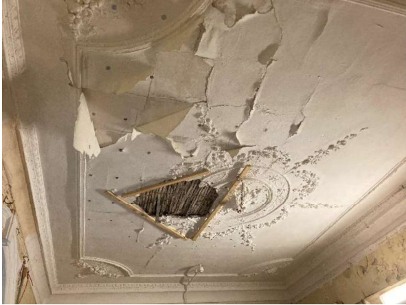
View of ceiling showing restraint works.
