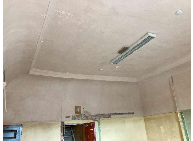
Coved detail similar to Room 2.06 but with extra run mould detail around the compartment.
