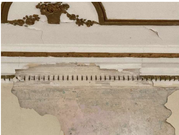
Dentil cornice detail.
