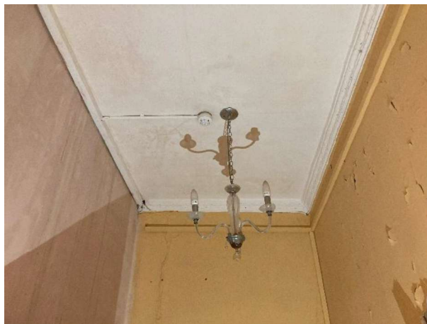
Landing ceiling with waterleaf detail to cornice.
