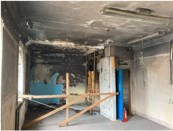
View of 2.01 looking towards landing.
