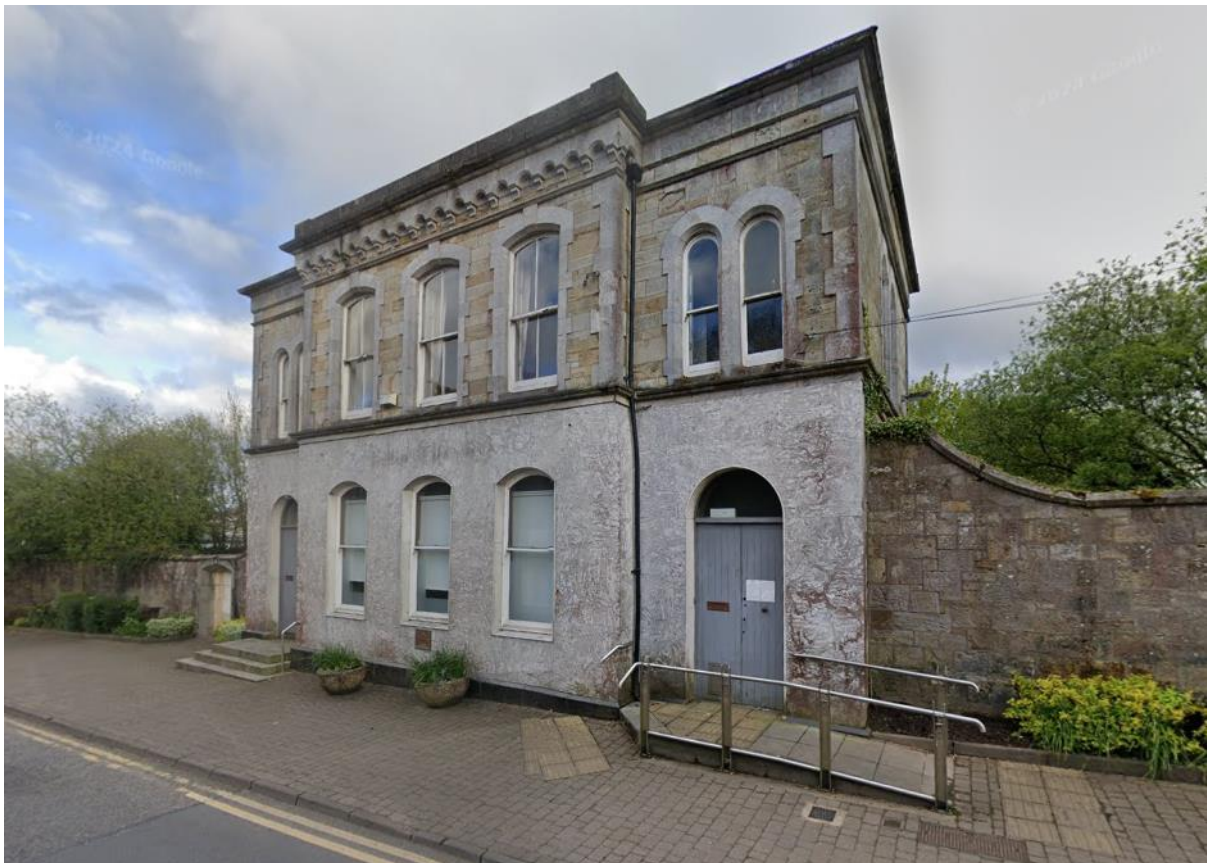
Former Bank of Ireland Building West Street, Lismore
