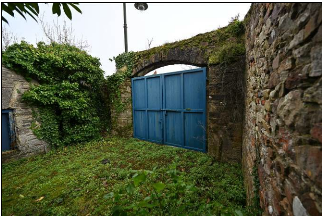
Photograph 7: Interior view of the vehicle entrance, looking east.
