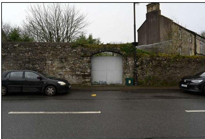
Photograph 3: View of coach gate entrance from New Street, looking west.
