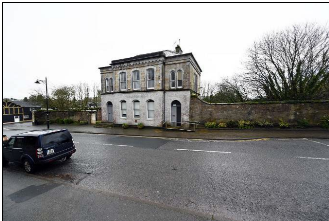
Photograph 1: Street front elevations of the development site, the former Bank of Ireland building, looking south.
