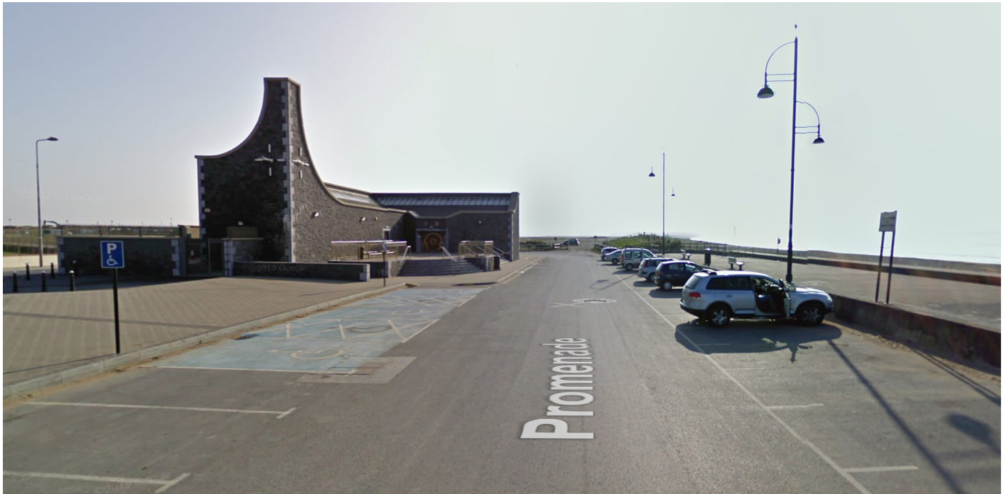
Fig.3; view of lower promenade and existing public toilets building
