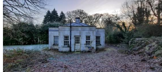
Rear elevation of the Middle Gate Lodge
