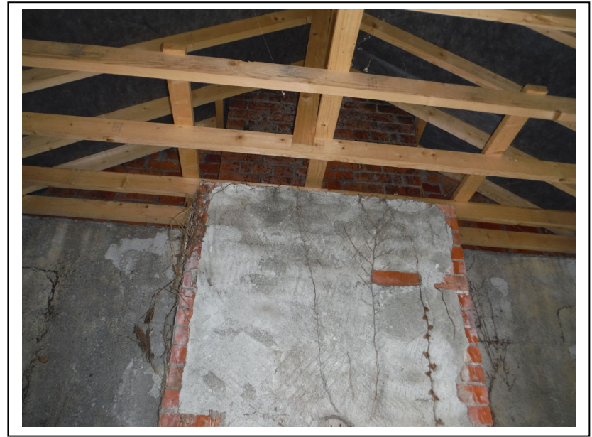
Fig 18 New Roof structure
