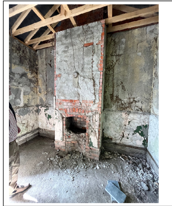
Fig 16 Fireplace in ladies toilet
