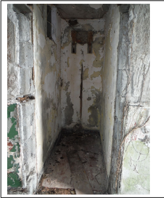
Fig 17 WC Recess in ladies Toilet
