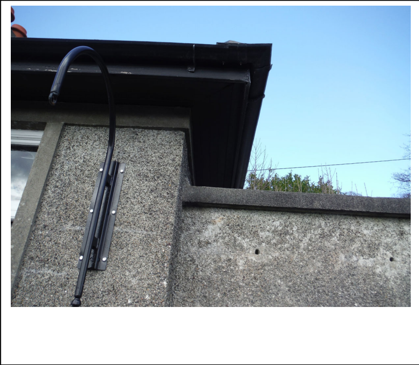
Fig 9 New renovation Eaves with Timber fascia soffit and new metal Gutter
