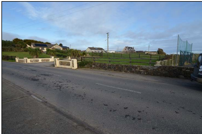
Photograph 1: Point at which the Relief Road will meet the R673; looking east.
