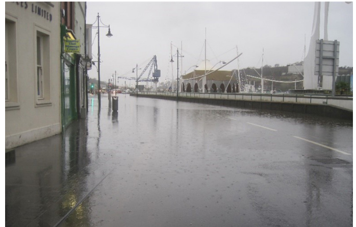
Figure 12: Flooding on the Quay Waterford City, February 2014.
