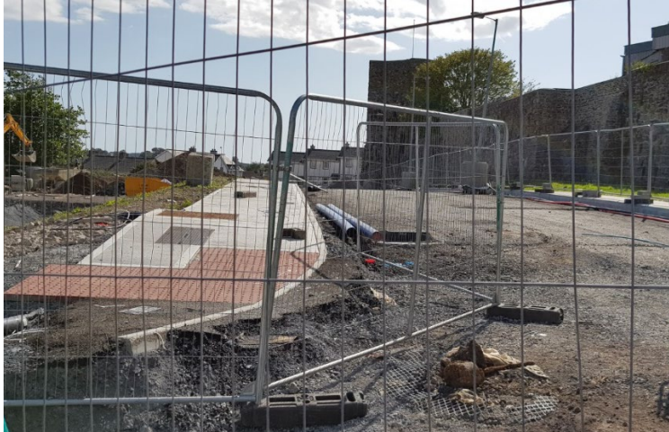
Image 5.10: Brown's Lane road improvements
